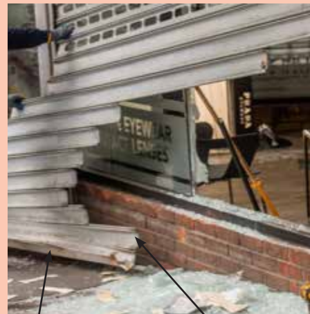
No end locks makes slats easier to slide out
